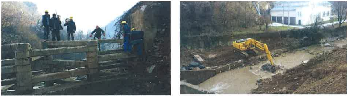
Fig. 3. Check-dams on the Pena River after the flash floods on 3 August 2015 and ongoing reconstruction
